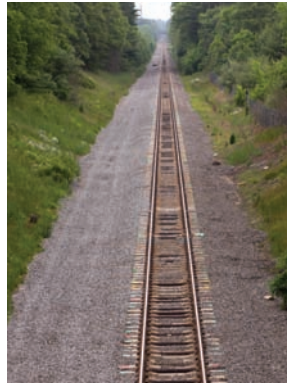
Bottom right, looking south from a bridge at Plymouth Street in Middleborough: Wooden ties are used to shore up sections of track where deteriorating concrete ties could create problems for trains, which travel up to 70 miles per hour on the straightaway. The green, yellow, and white paint on the ties indicate those that need to be replaced or monitored. Bottom left: New concrete ties await installation at a staging area in South Bridgewater. In the background are scores of wooden ties ready to be placed in problem areas until the broken concrete ties can be removed and replaced. Top left: A close-up photo shows dozens of consecutive ties, painted to mark them as defective, in various stages of distress. There are cracks, breaks, and detached chunks of concrete.
